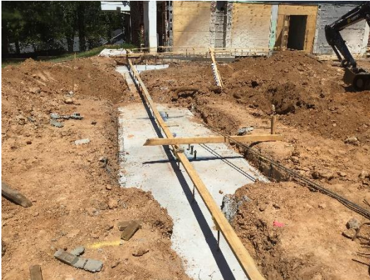
Building Foundation and Anchor Bolts
