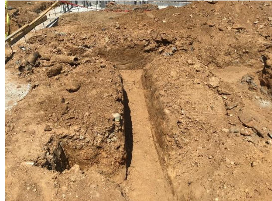
Excavating for Underground Plumbing
