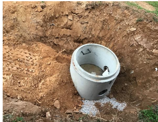
Sanitary Sewer Structure Installation
